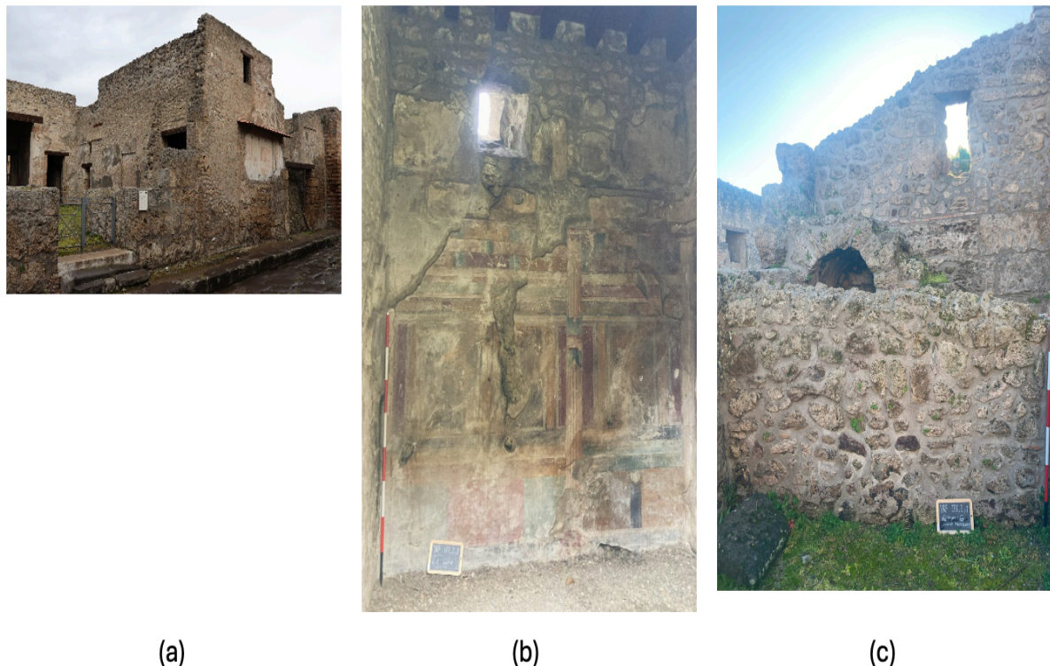
Figure 2. Current state of the House of Trebius Valens (III, 2, 1) and some of its remaining window openings. (a) The façade of the house and the southern wall of triclinium d with a clerestory window; (b) western inner wall of cubiculum l and its wall painting with a small splaying window (photograph by Henna Ala-Lehtimäki); (c) western inner wall and a window opening of corner room h seen from room g (photograph by Henna Ala-Lehtimäki).
